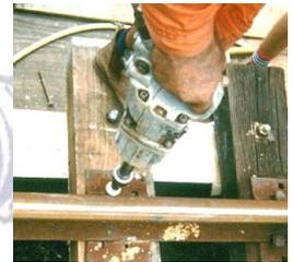
**2) SEMI-AUTOMATED:** Standard pedestrian style push along rail machines can be used to insert screws in an easy and much safer way.
